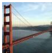
The Golden Gate Bridge (USA)
