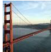
The Golden Gate Bridge (USA)
