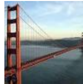
The Golden Gate Bridge (USA)
